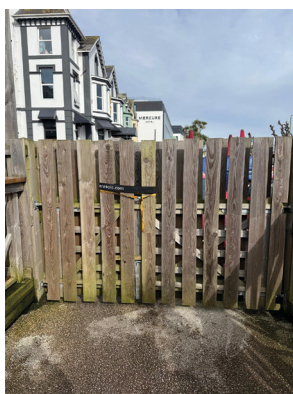
Evidence of side gate to Kernou road, secured at 01.00am.
